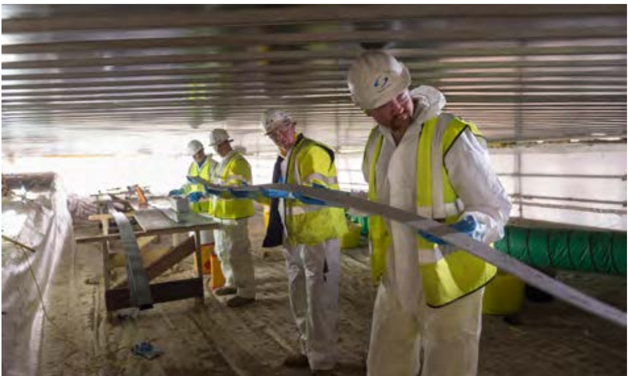
Installation of Sika® CarboDur® carbon fibre plates.
