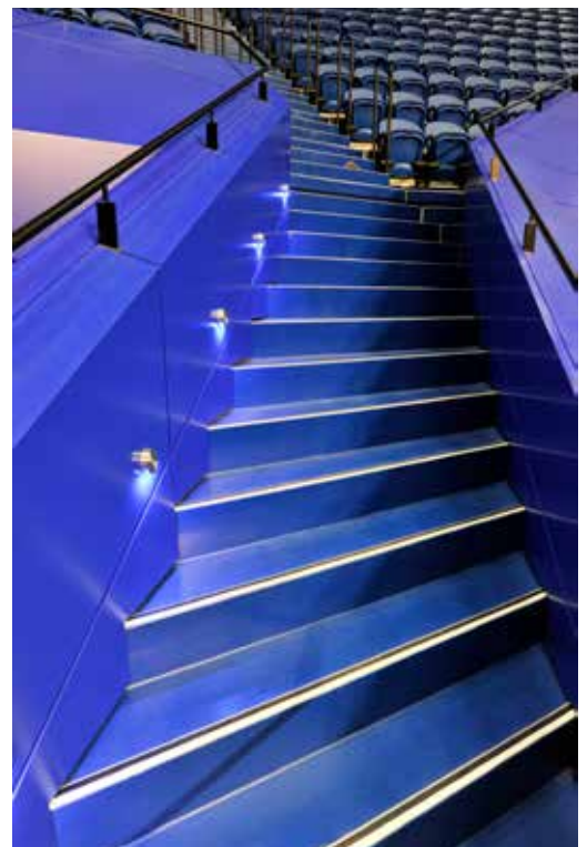
Sikafloor®-2530W coating was specified and used on all concrete seating platforms, associated stairs and access ways within the stadium area.
