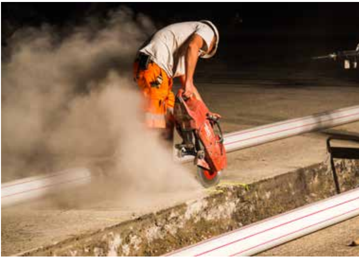
Detail work in tough conditions.
