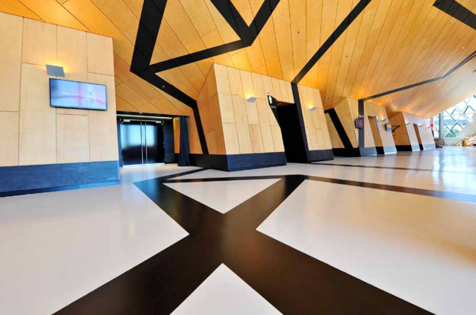
As with most new stadiums, floors play an important part of the durability and overall design considerations.
