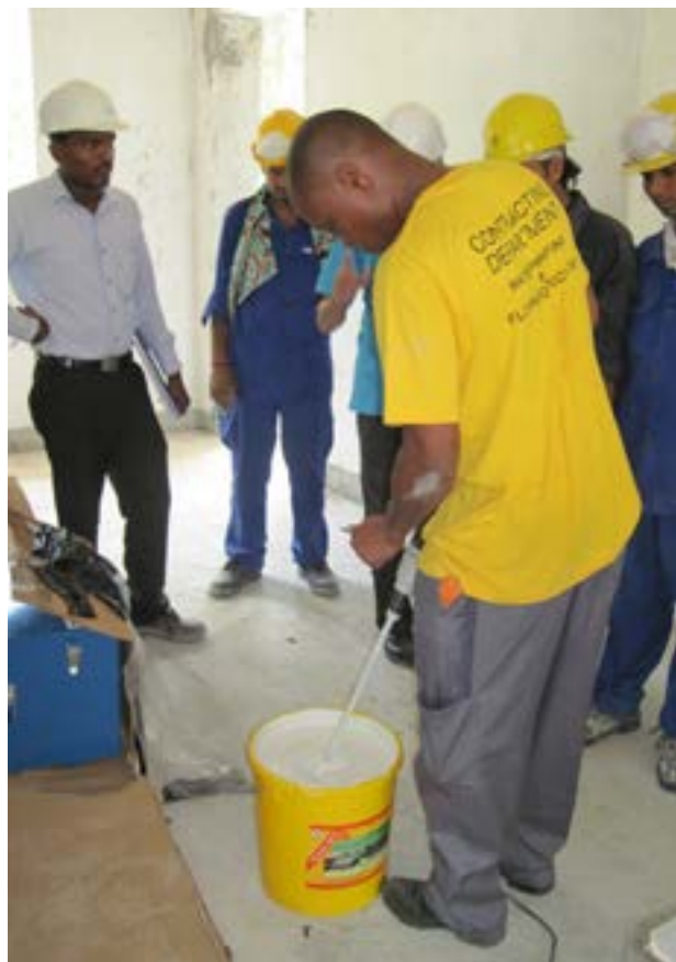
Training with Sikalastic 850W at the construction site
