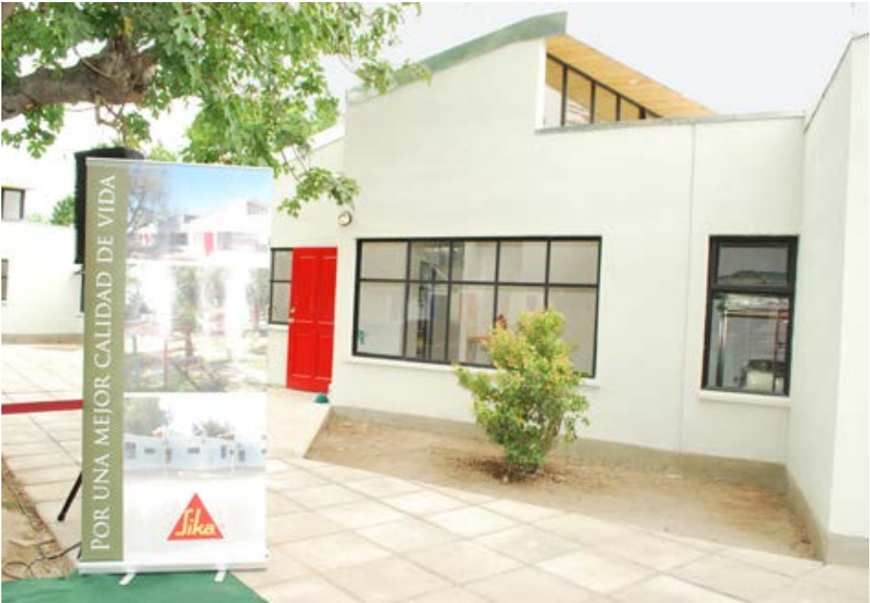
View of the new building of John XXIII Home, Coanil
