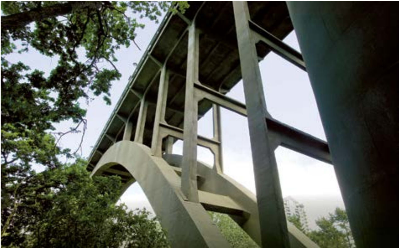
Auckland's Grafton Bridge, the world's largest single span reinforced concrete arch bridge when constructed in 1910, has continued its history of innovation by using Sika CarboShear technology in its 2010 strengthening. Sika CarboDur® plates provide flexural and shear strengthening
