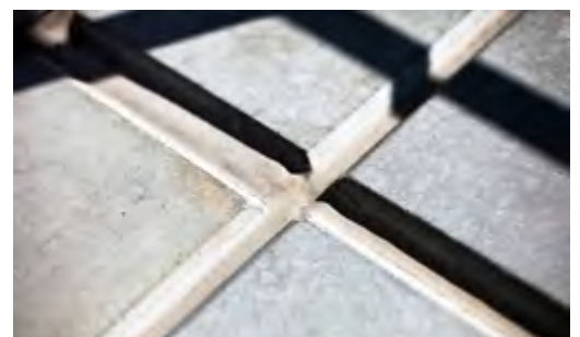
Joint sealing with Sikadur-Combiflex® between the precast reinforced concrete elements.
