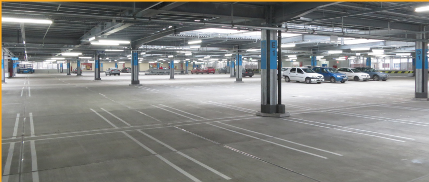
Lot de parcare, București, România | Concrete car park deck in Bucharest, Romania
