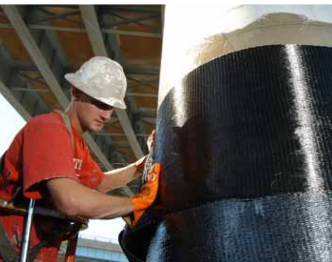
Usage of SikaWrap®-600 C and Sikadur®-300
